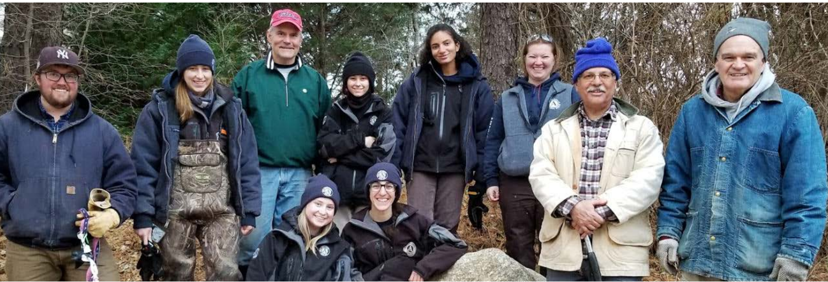
AmeriCorps Members and DCLT Stewardship Volunteers pose after installing a boardwalk at Cole's Pond Bog. (Photo by Tyler Maikath)
